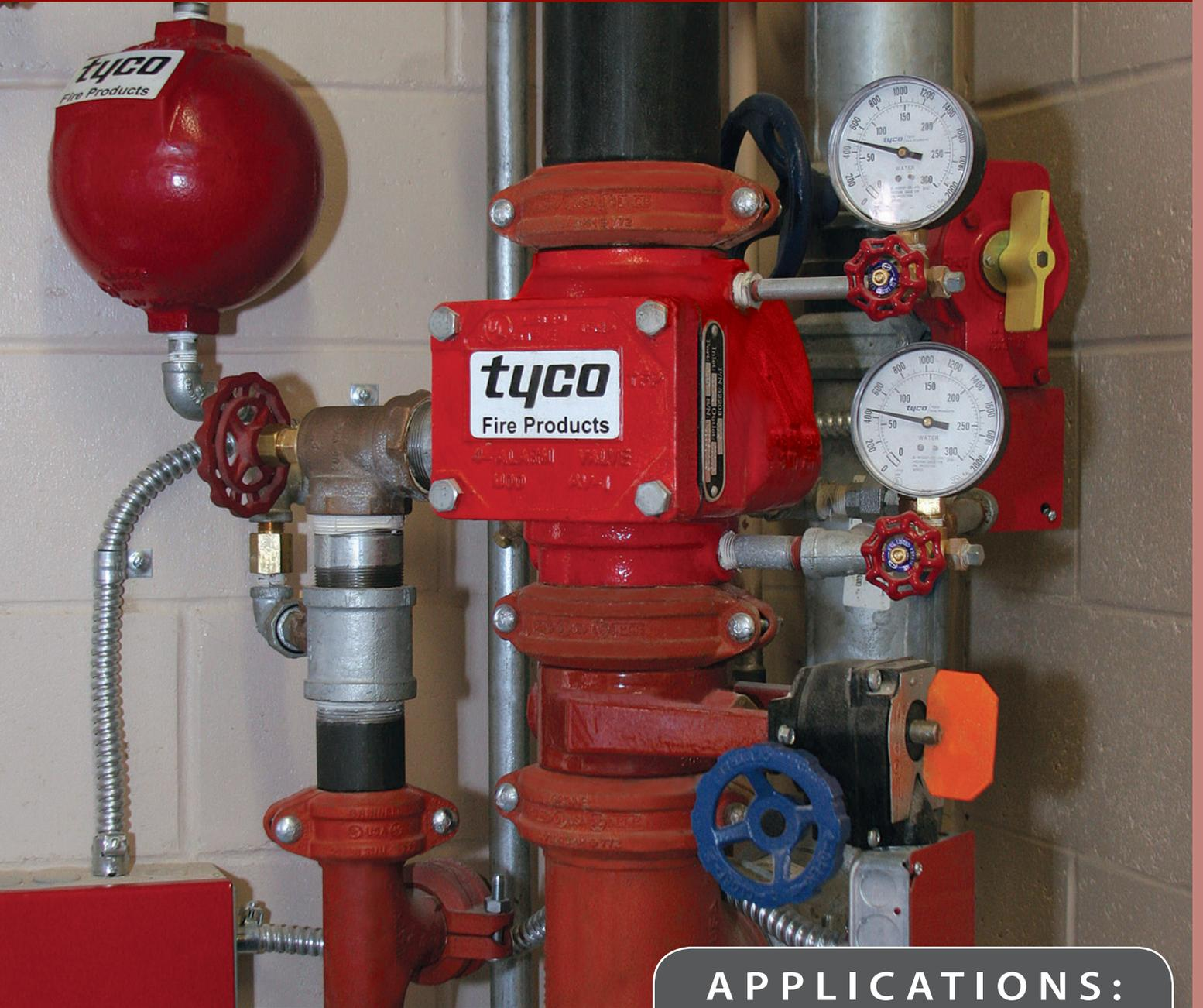
**Wet Pipe Sprinkler Systems** are designed for use in applications where the temperature is maintained above freezing. In such systems, the entire piping network is fully pressurized so that water is discharged from a sprinkler head immediately after actuation.
