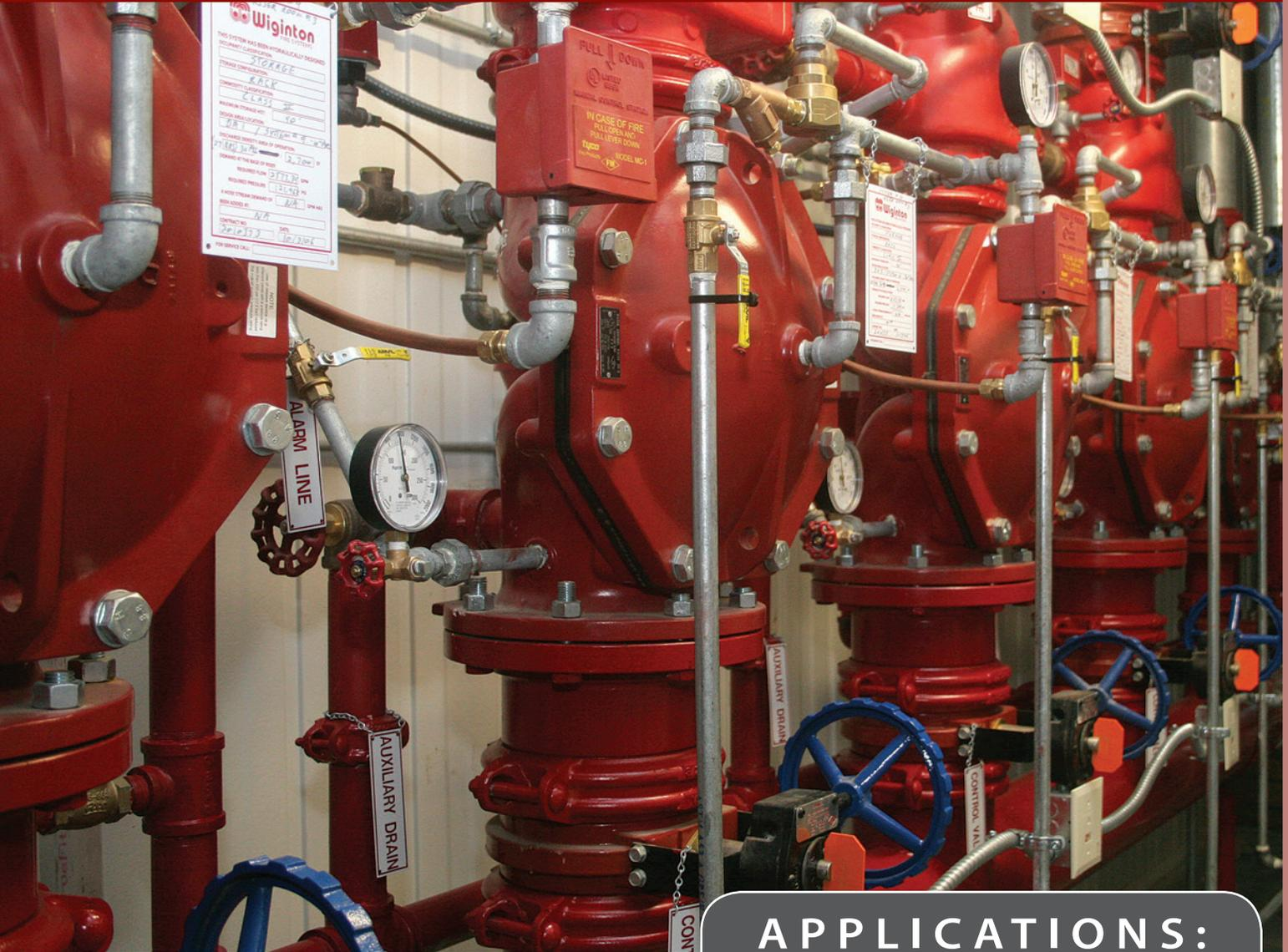
**Deluge Systems** are normally used in special hazard installations where water must be applied to an entire area for protection. They use open sprinklers or spray nozzles attached to a piping system connected to a water supply through the deluge valve. The deluge valve is used to control water flow into deluge, preaction, and special types of fire protection systems in response to a fire. This valve is opened by a fire detection system installed in the same areas.
