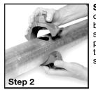
**Step 2.** With one nut and bolt removed, swing the coupling around the pipe as shown.
