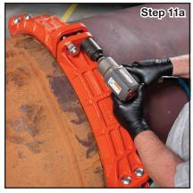
**Step 11.** Tighten all nuts uniformly to the recommended bolt torque. (Refer to Figure 1.) Ensure that the coupling key aligns with the grooves on both pipes when tightening the nuts.
