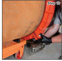
**Step 9.** Attached three more coupling segments using two bolts and nuts for each connection between the segments. Loosely tighten the nuts.
