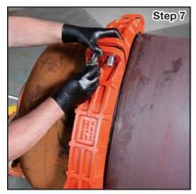
**Step 7.** Slide the coupling segment so that the coupling segment end is centered on the pipe and attach a second coupling segment to the first using two bolts and nuts. Loosely tighten the nuts.
