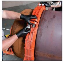
**Step 8.** Slide the assembled coupling segments so that the newly installed segment is centered to the pipe. This allows the pipe to support the coupling weight as it is being assembled. Attach a third coupling segment using two bolts and nuts. Loosely tighten the nuts.
