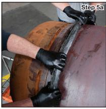
**Step 5.** Bring both pipes together, ensure proper alignment, and roll the gasket over into position. Ensure the gasket is centered between the
