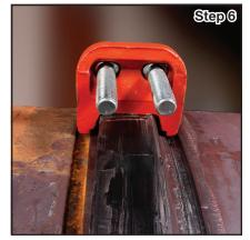
**Step 6.** Set the first segment of the coupling over the gasket and ensure the coupling keys align with the grooves on both pipes.
