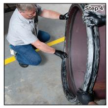
**Step 4.** Install the gasket by placing it over the end of the first pipe section. Ensure that the gasket is aligned with the outer edge of the groove (closet to the end of the pipe).
