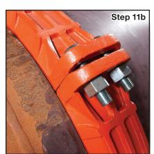
**CAUTION** Failure to ensure proper alignment of the coupling keys with the pipe grooves may result in equipment failure and/or personal injury.
