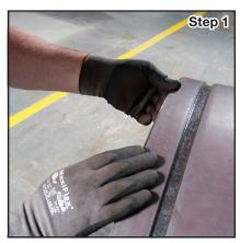
**Step 1.** Inspect exterior groove and ends of the pipe to verify all burrs, loose debris, dirt, chips, paint and any other foreign material such as grease are removed. Pipe end sealing surfaces must be free from sharp edges, projections, indentations, and/or other defects.
