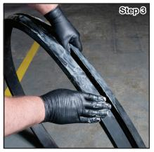
**Step 3.** Roll the gasket inside-out and cover the gasket with a fine layer of lubricant. To prevent deterioration of the gasket material, a petroleum lubricant should never be used on Grade "E" "EPDM. For assembly below 40°F (4°C), a petroleum-free silicone lubricant must be used to prevent freezing of the lubricant.
