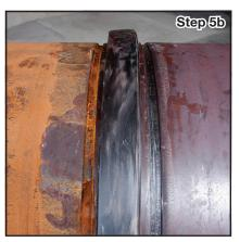
grooved portions of each pipe. The gasket should not protrude into the grooves on either pipe segment or extend beyond the pipe ends.
