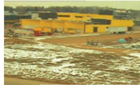
GlenOak High School and Community Center Winter Construction
