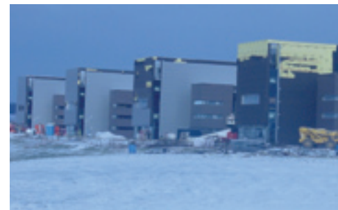
GlenOak High School and Community Center Near Completion
