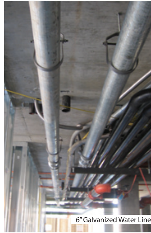
6" Galvanized Water Line
